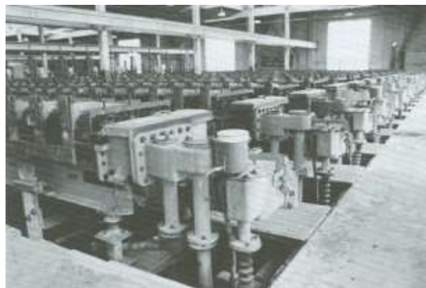
ICI Mercury Cell room, Cornwall.
