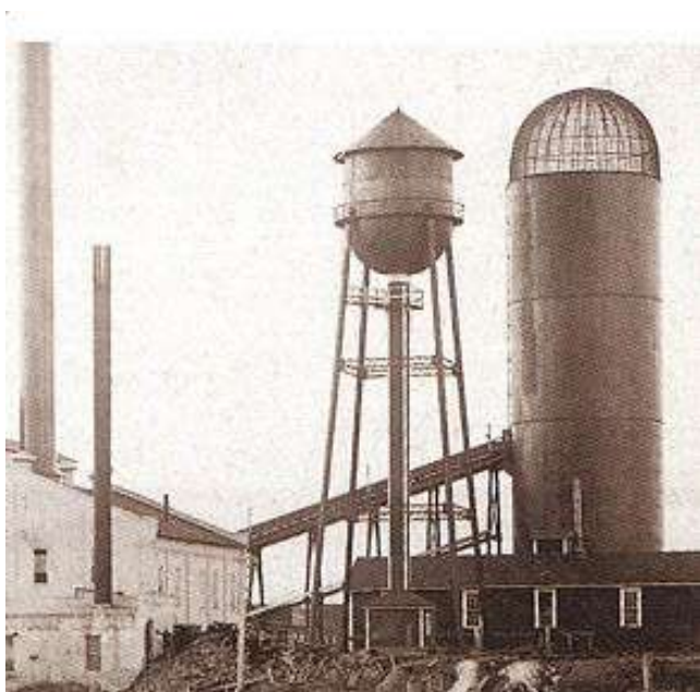
Figure 8: Sawdust burner at Rainy River Mill, 1910.
