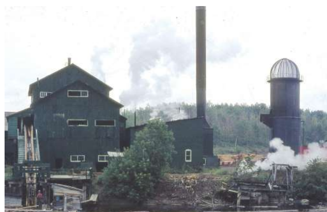
Figure 9: Sawdust burner at sawmill located at Field, Ontario, 1976.
