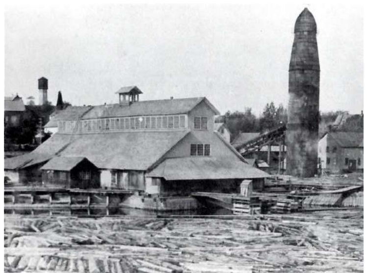
Figure 5: Sawdust burner at Parry Sound Lumber Company, Parry Sound, 1900.
