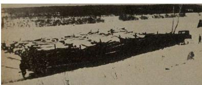
Sleds loaded with pulpwood being hauled by Holt 10-Ton, from the Canada Lumberman.
