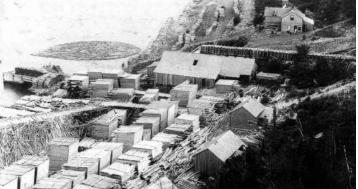
The flume carried logs down to Lymburner's mill; offshore, a raft of logs.
