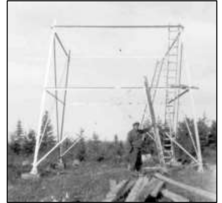
Fire tower 3: Gin pole to the right of the main support pole.
