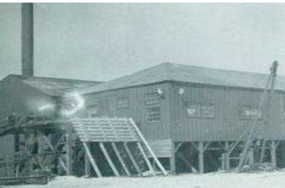
The front end of the Kenesis Lake mill showing the jack ladder.
