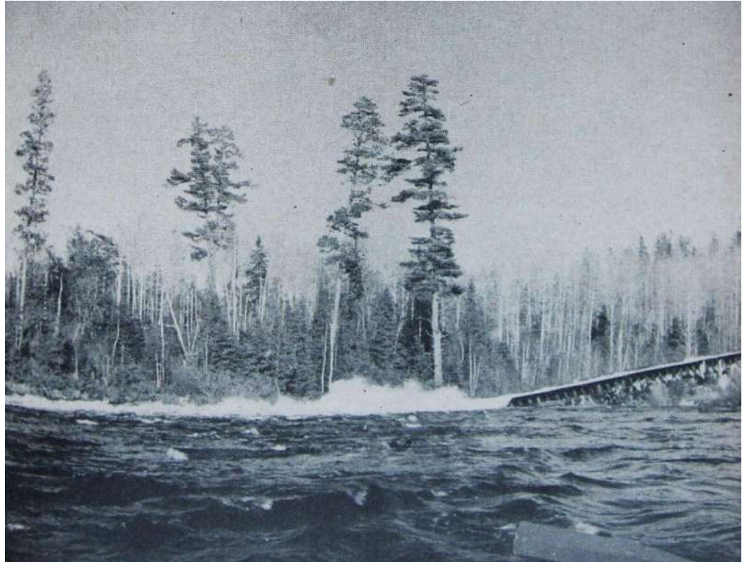
The flume – a spectacular method used to transport logs overland. K.M. Andresen
