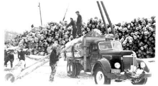
Loading veneer logs on a truck with a jammer.
