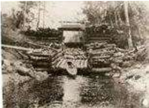
The anatomy of a logging dam is exposed in this photo, taken in the early 20 th century on Caribou Creek in the Pickerel River watershed. Timber cut nearby and shaped with crosscut saw and broad axe formed the components, and rock-filled cribs hold it all in place (Photo Credit George Knight)
