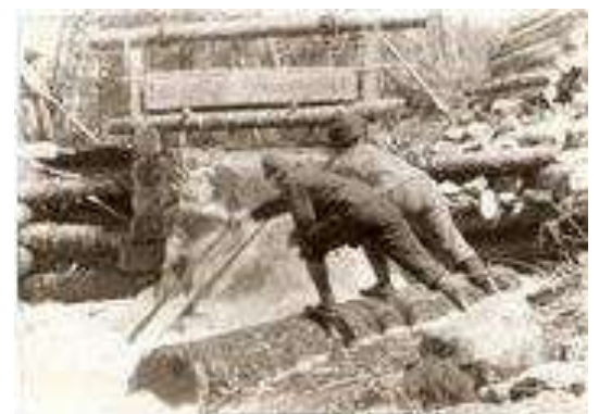
The topmost stop log has been lifted, allowing saved water to start logs on the journey down the sawmill. The creek is tributary to the Pickerel River, in northern Parry Sound District (Photo Credit: George Knight)
