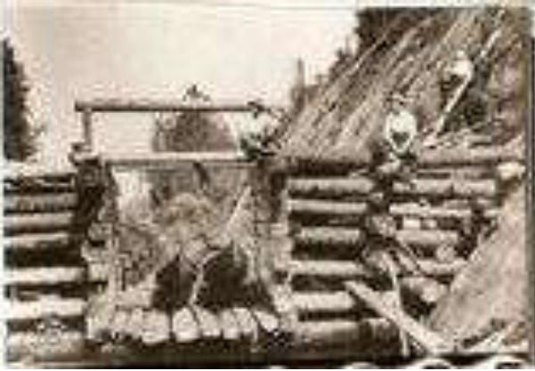
This dam, on Four Bears Creek, a tributary of the Magnetawan River, shows how lumbermen harnesse small streams to drive sawlogs. Here, in midsummer, the watercourse is nearly dry (Photo courtesy of Roy Smith)
