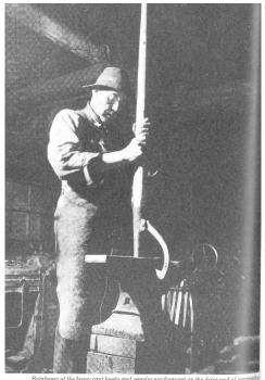
Breakages of the heavy cant hooks and peavies are frequent on the drive and of necesare kept in constant repair.  $K.\ M.\ Andre$
